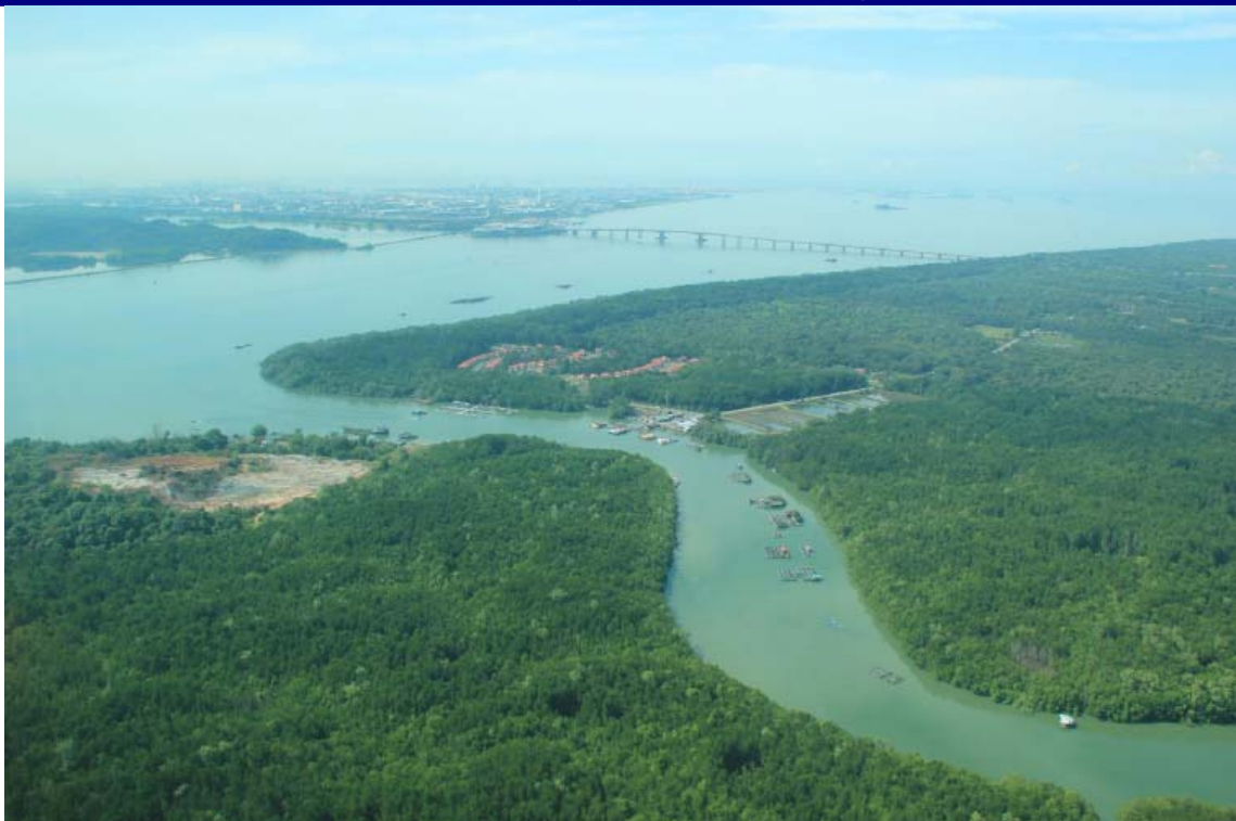
Figure 2: Helicopter view for the Pendas land – close proximity to the Second link to Singapore
